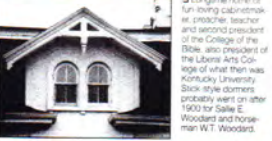
Longtime home of fun-loving cabinetmaker, preacher, teacher and second president of the College of the Liberal Arts College of what then was Kentucky University. Six-story dormers probably went on after 1900 for Sallie E. Woodard and horseman W.T. Woodard.
