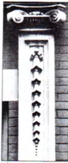
Chairs of hooks, or belfowers, decorate building listed as Ellis before Falls in 1903.
